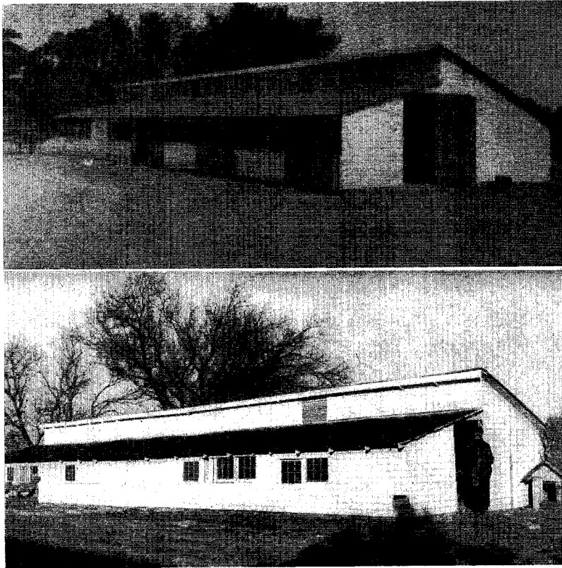
FIG. 3.—One of the few remaining semimonitor poultry houses as it appeared in 1926. The lower picture shows the same house in 1940. Note that the upper windows were removed and the front was boarded up. The windows were used to close the lower open front. This house, located in District 3, was built in 1923.
